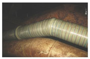
Technowrap<sup>™</sup> ULT (Ultra Low Temperature) repair system is the ideal solution for repair and strengthening of pipes where low ambient temperatures are an issue. The resin system has an enhanced curing rate at lower ambient temperatures.
