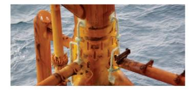
Technowrap Splashzone™ can be applied either on wet surfaces or within wet or submerged environments. The repair system consists of either a carbon or glass reinforcement encased in a water tolerant epoxy resin. Based on successful conclusion of the qualification tests (according to ISO 24817) and application trials, the Technowrap Splashzone™ repair product can provide a repair solution for a design lifetime of up to 20 years.
