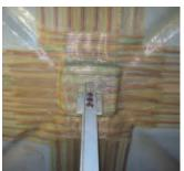
Technowrap Potable Water<sup>™</sup> is a design engineered glass-based repair system specifically designed and certified for potable water applications and can be used on all pipe work components. It consists of a glass fibre reinforcement encased in an epoxy resin which has been specifically formulated for use in drinking water applications. The repair system has been successfully tested to BS 6920, confirming its suitability for potable water applications.
