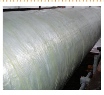
Technowrap PRS<sup>™</sup> (Pipeline Repair System) is a composite repair system specifically for long, straight piping sections or pipelines. It was developed in response to demand from clients who required a product that provided a cost-effective method of returning externally corroded pipelines to their original pressure retention capability and structural design integrity.
