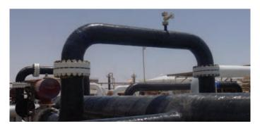
Technowrap H.P. PRS<sup>™</sup> (High Pressure Pipline Repair System) has been designed for use on land. The system's intended application is for large diameters of pipe work, such as a 36 inch pipe operating at 50 bar pressure, and is ideally suited to the Middle East market. The unidirectional carbon based cloth applied with our epoxy resin system results in a fast application time.
