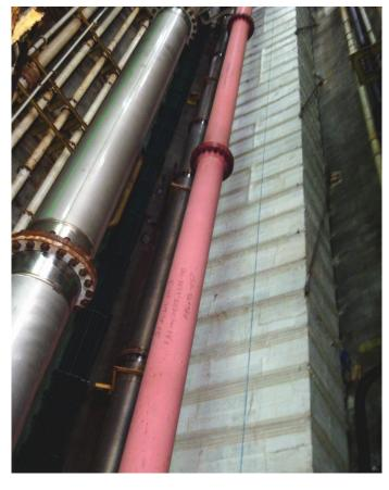
Technowrap™ E1 is an external corrosion protection coating developed for pipework and structures.
